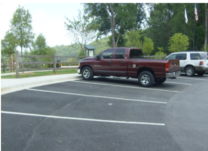
Porous asphalt used at a metro Atlanta area parking lot
