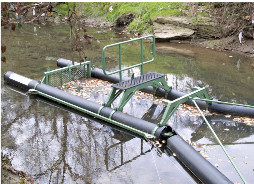
Figure 18: Left - Bandalong in Proctor Creek Figure 19: Right - "boom style" trash trap in Anneewakee Creek
