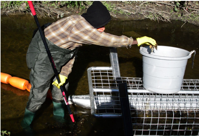
Figure 11: Litter Gitter cleanout
