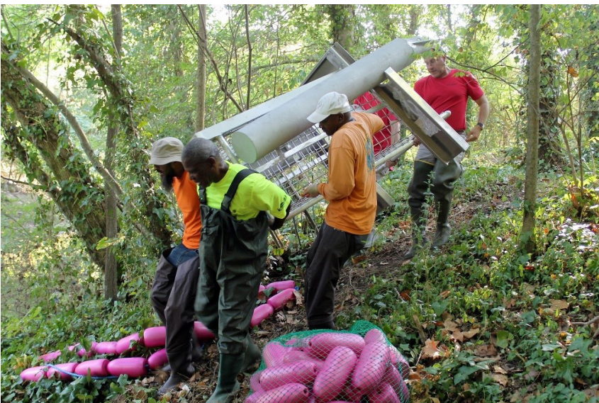
Figure 5: Aluminum Litter Gitter installation at Maddox Park
