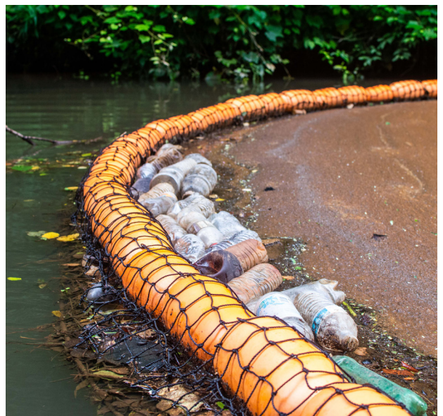
Figure 18: Left - Bandalong in Proctor Creek Figure 19: Right - "boom style" trash trap in Anneewakee Creek
