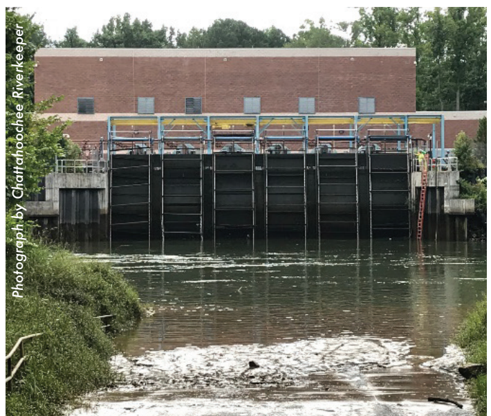
One of two dozen raw water withdrawal intakes on the Chattahoochee River, its lakes and tributaries that are necessary for communities' clean drinking water.
