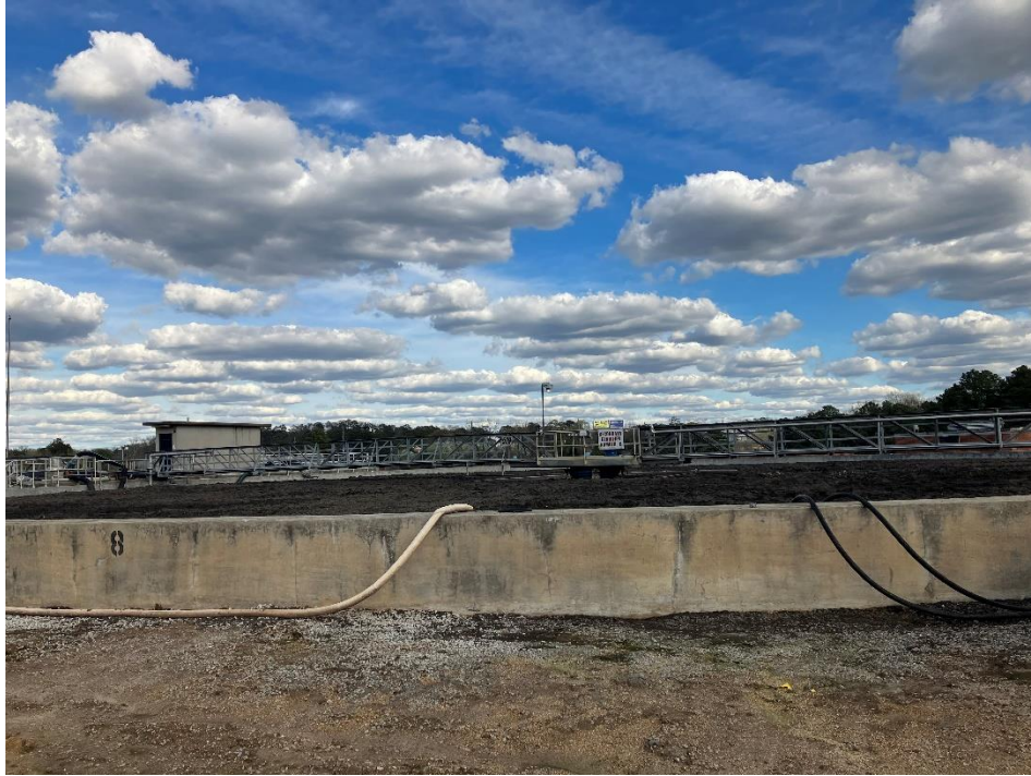
SC Photo 8: Secondary Clarifier #8
