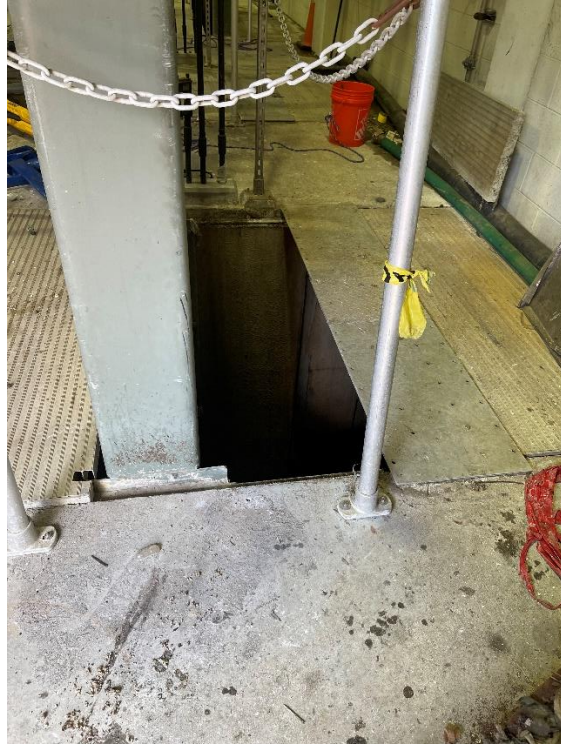
O&M Photo 1: Open Space on the Bar Screen
