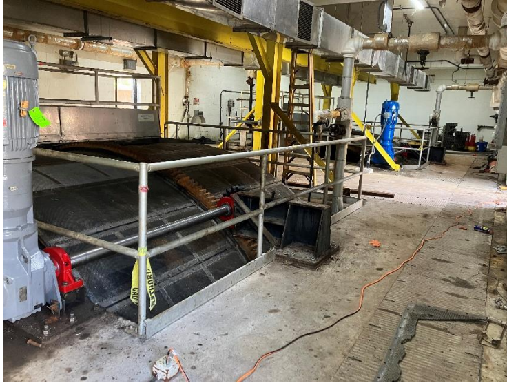
Preliminary Screening Photo 2: Drum Screens
