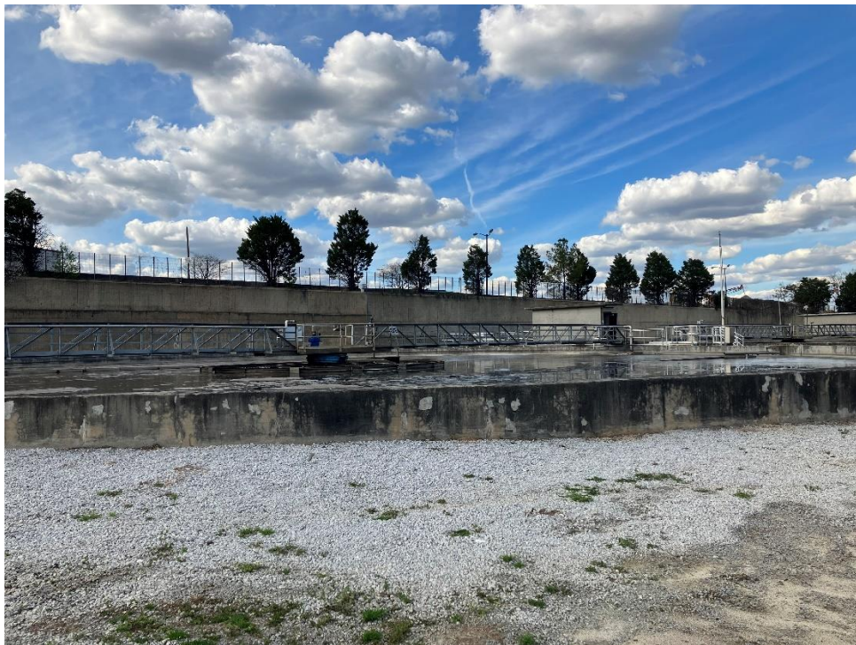
SC Photo 7: Secondary Clarifier #7
