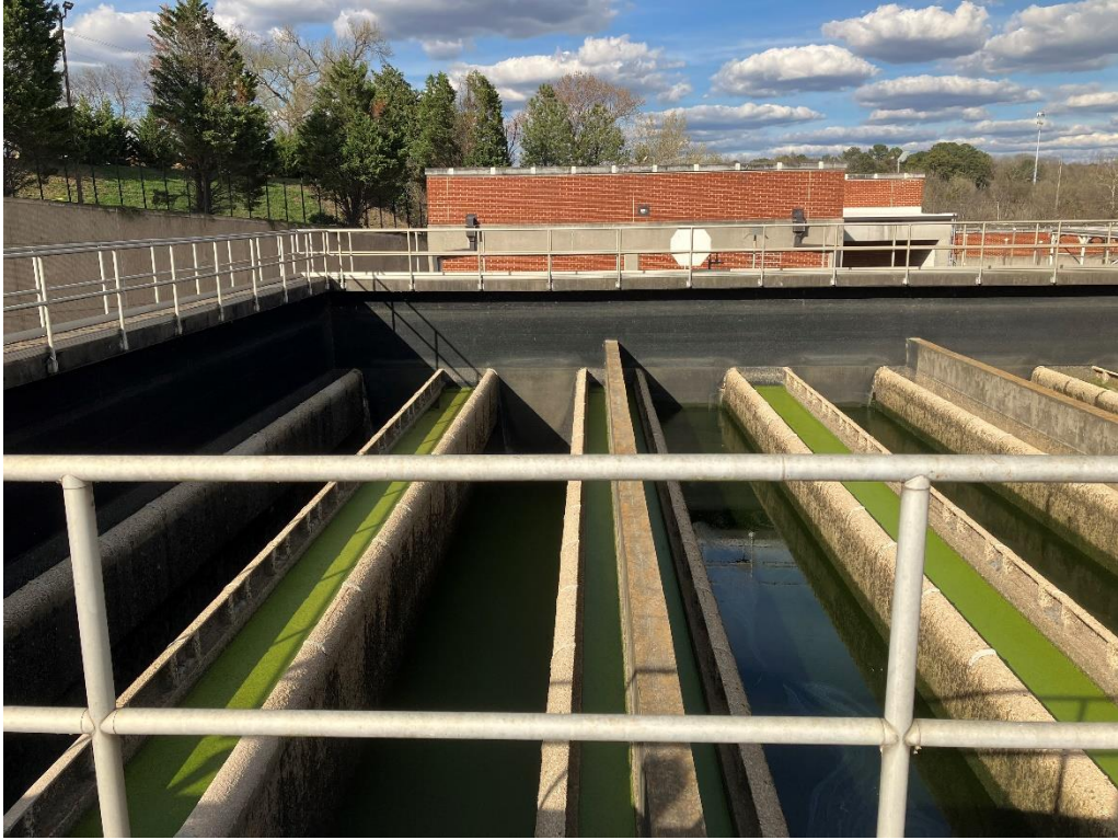
Tertiary Treatment Photo 7: Offline Sand Filters (1)
