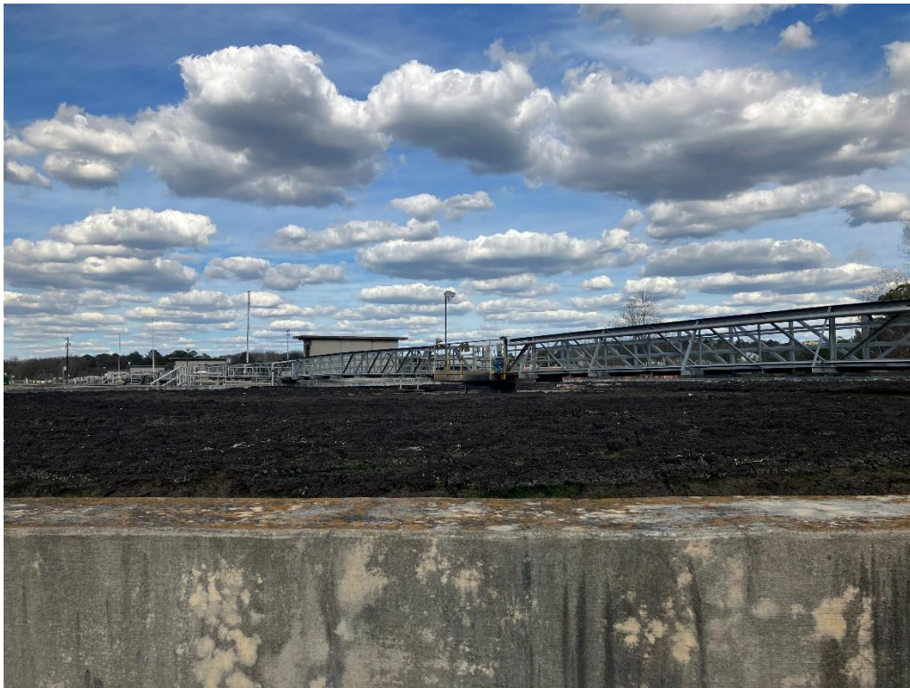
SC Photo 2: Secondary Clarifier #4
