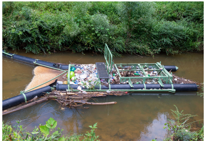
Large Storm Water Systems "Bandalong" trash trap in north Georgia
