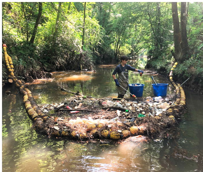
Watergoat INC “Watergoat” trash trap during cleanout in north Georgia
