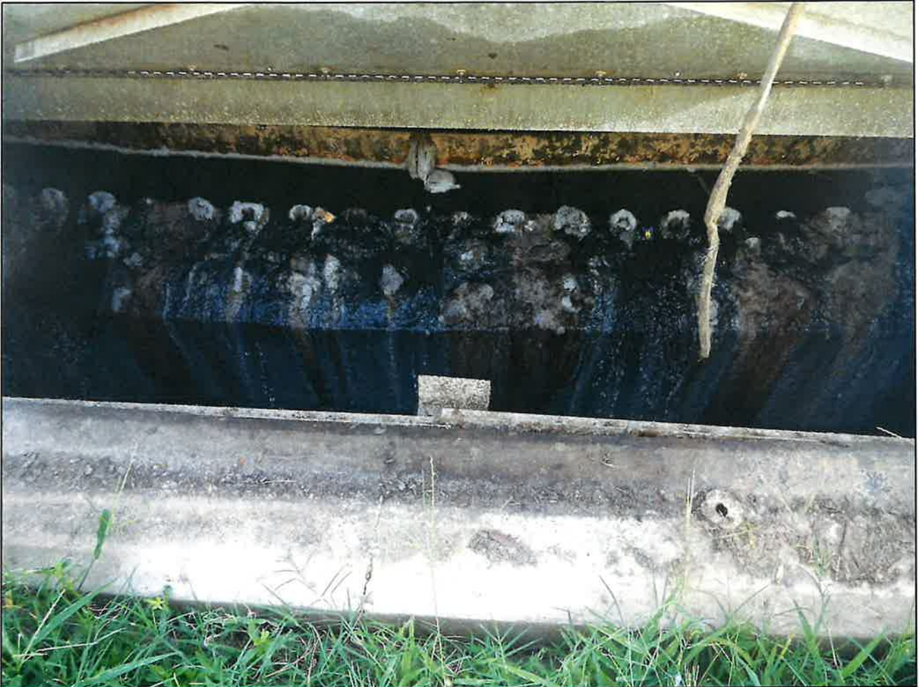
Photo 5. Primary Clarification – Debris and algal buildup on weirs, and evidence of solids passage over weirs; pictured is primary clarifier #8.
