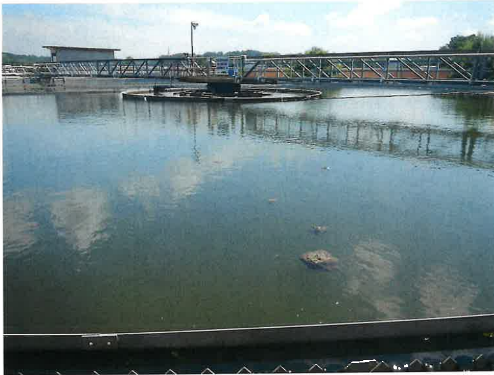
Photo 27: Secondary Clarifier #6 (picture provided by EPA)
