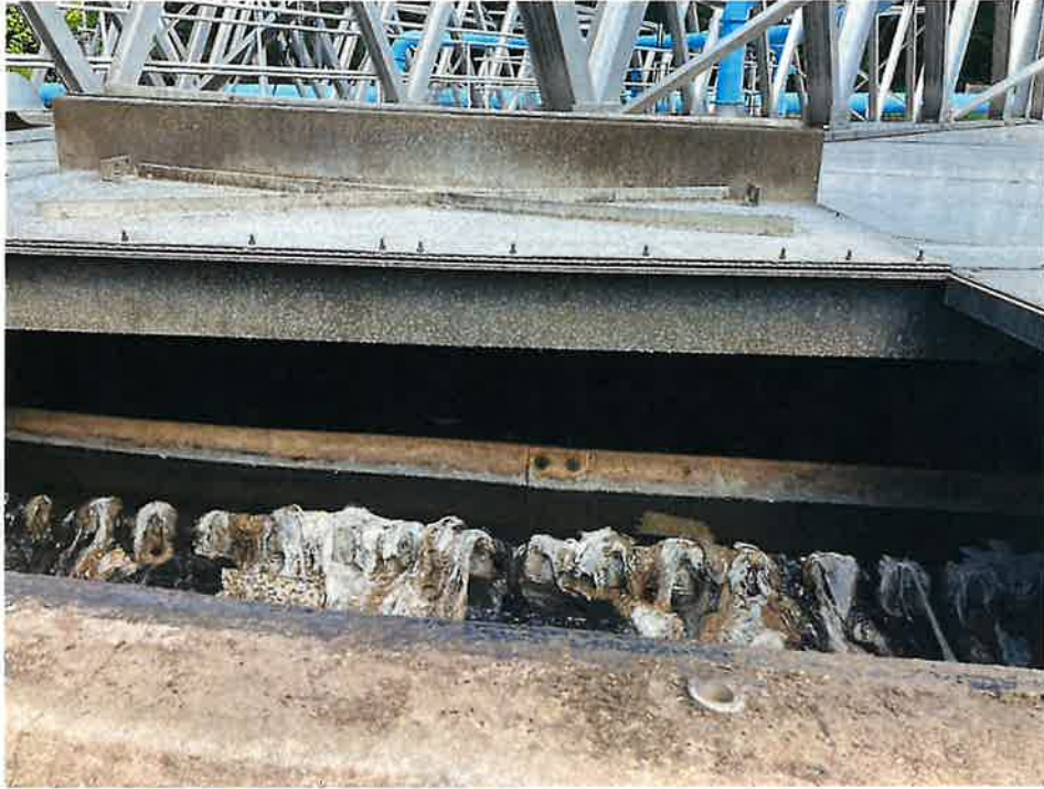
Photo 15: Primary Clarifier Weir (2)
