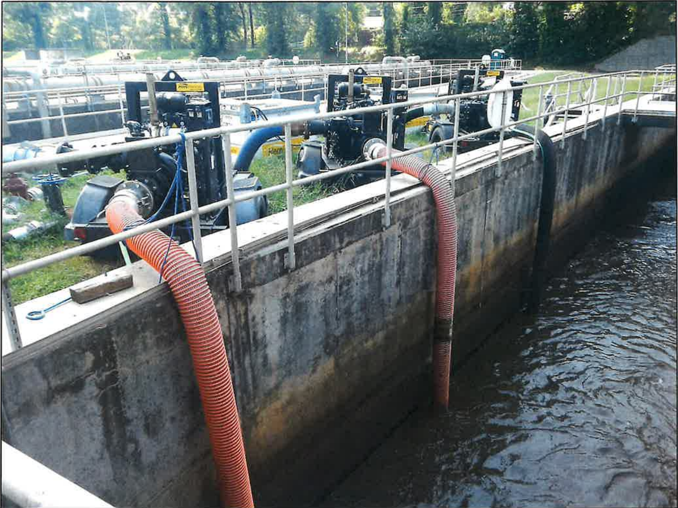
Photo 8. Mixed Liquor Pump Station Well – Bypass pumps in place.
