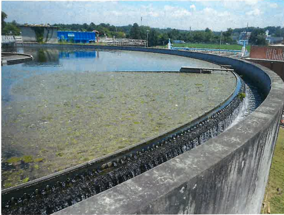
Photo 29: Secondary Clarifier #10 (picture provided by EPA)
