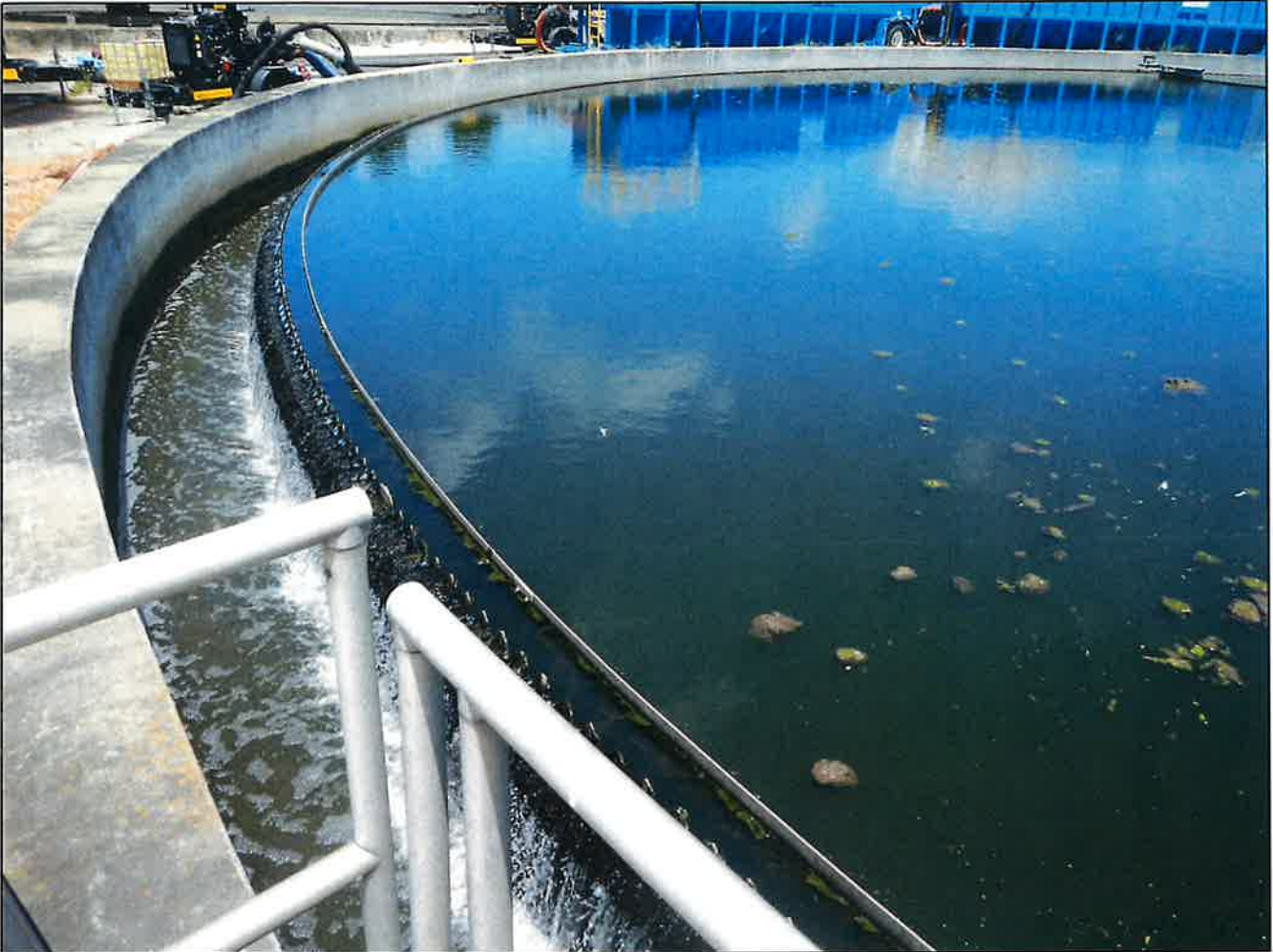
Photo 18. Secondary Clarification – Clarifier #10 with abundant floating solids and effluent channel with turbid effluent.
