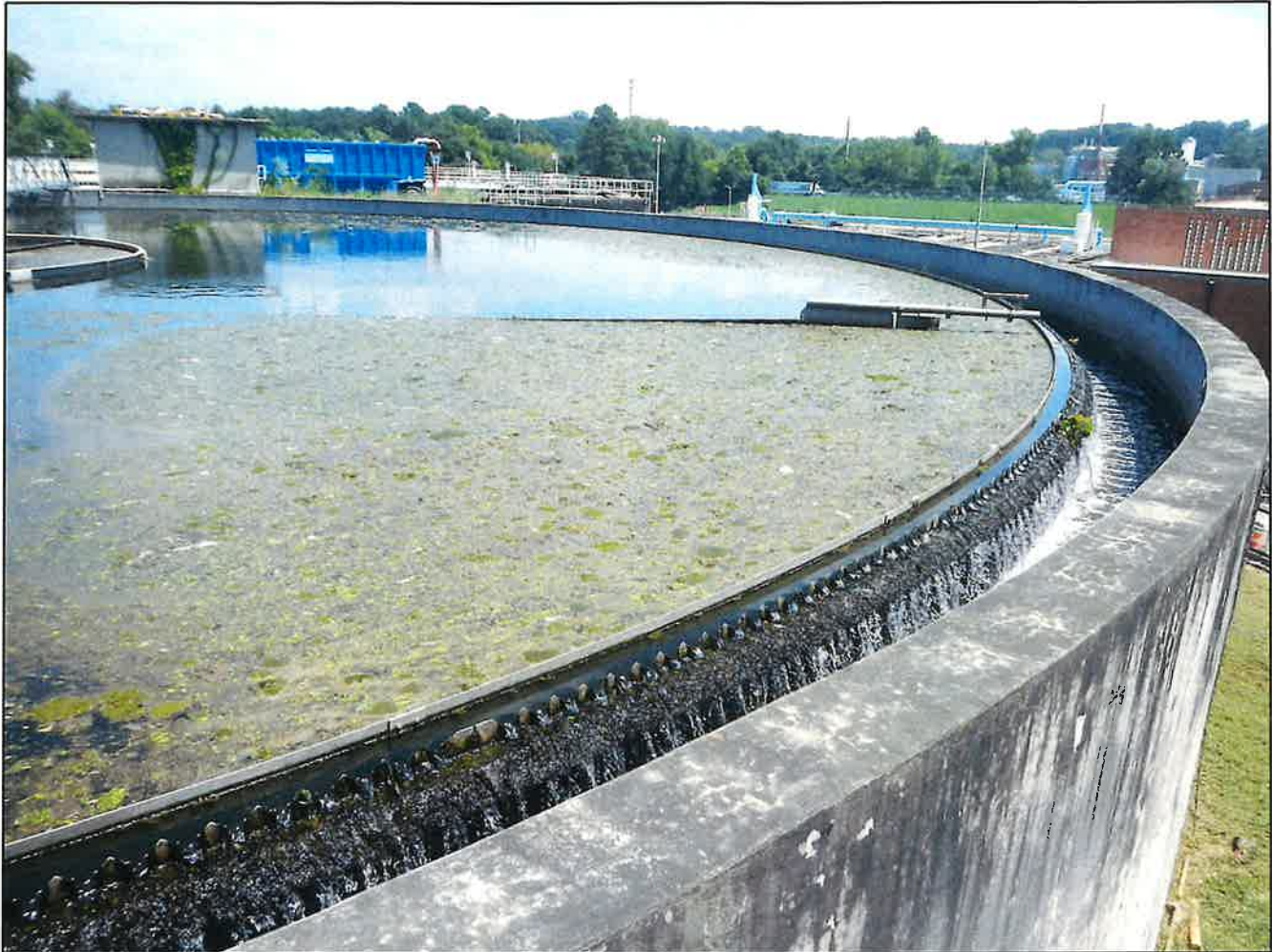
Photo 16. Secondary Clarification – Clarifier #10 in operation with floating solids blanket covered with plant life, and with abundant algal growth built up on the weir and effluent channel.
