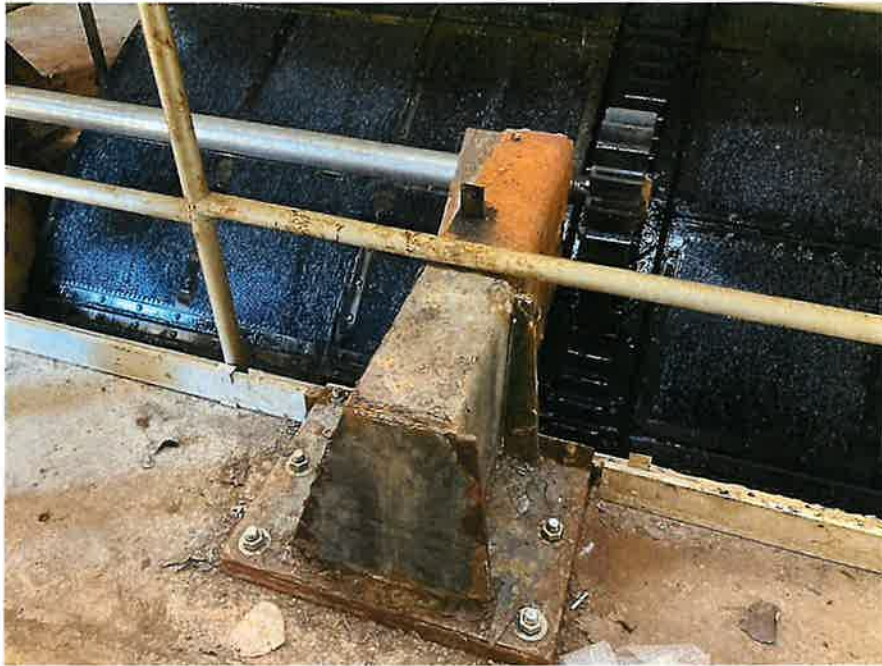
Photo 11: Motor Cover for Drum Screen #2
