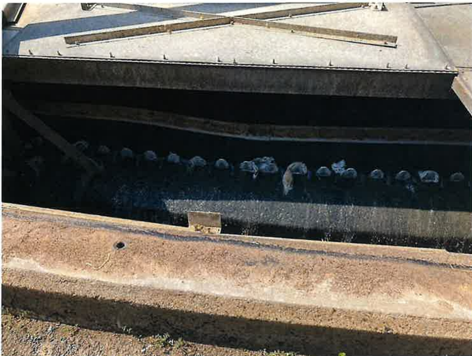
Photo 16: Primary Clarifier Weir (3)
