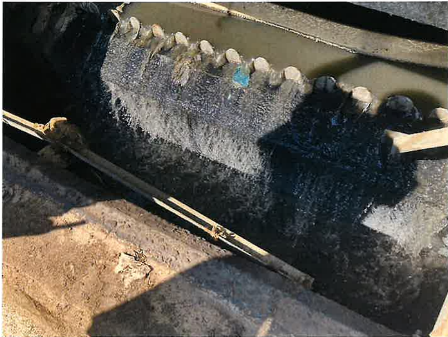
Photo 14: Primary Clarifier Weir (1)
